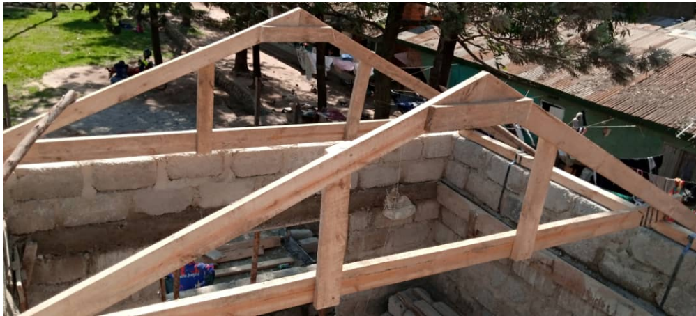
Fig. 21: Assembling Roof Trusses
