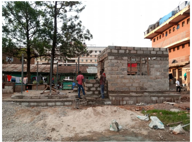
Fig. 18: Over Beam Walling
