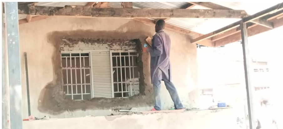
Fig. 26: Finishes around windows
