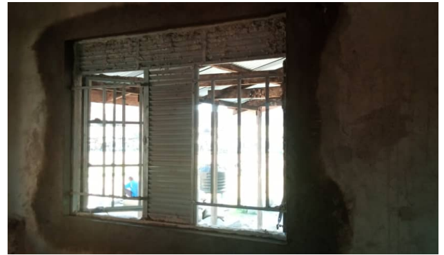
Fig. 24: Installation of Windows
