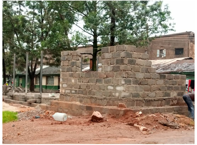
Fig. 16: Super Structure Walling
