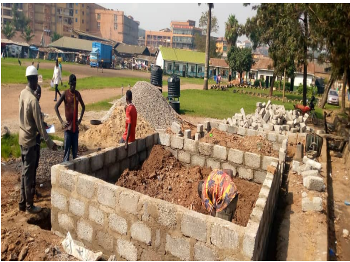
Fig. 7: Construction of Foundation (plinth) Walls
