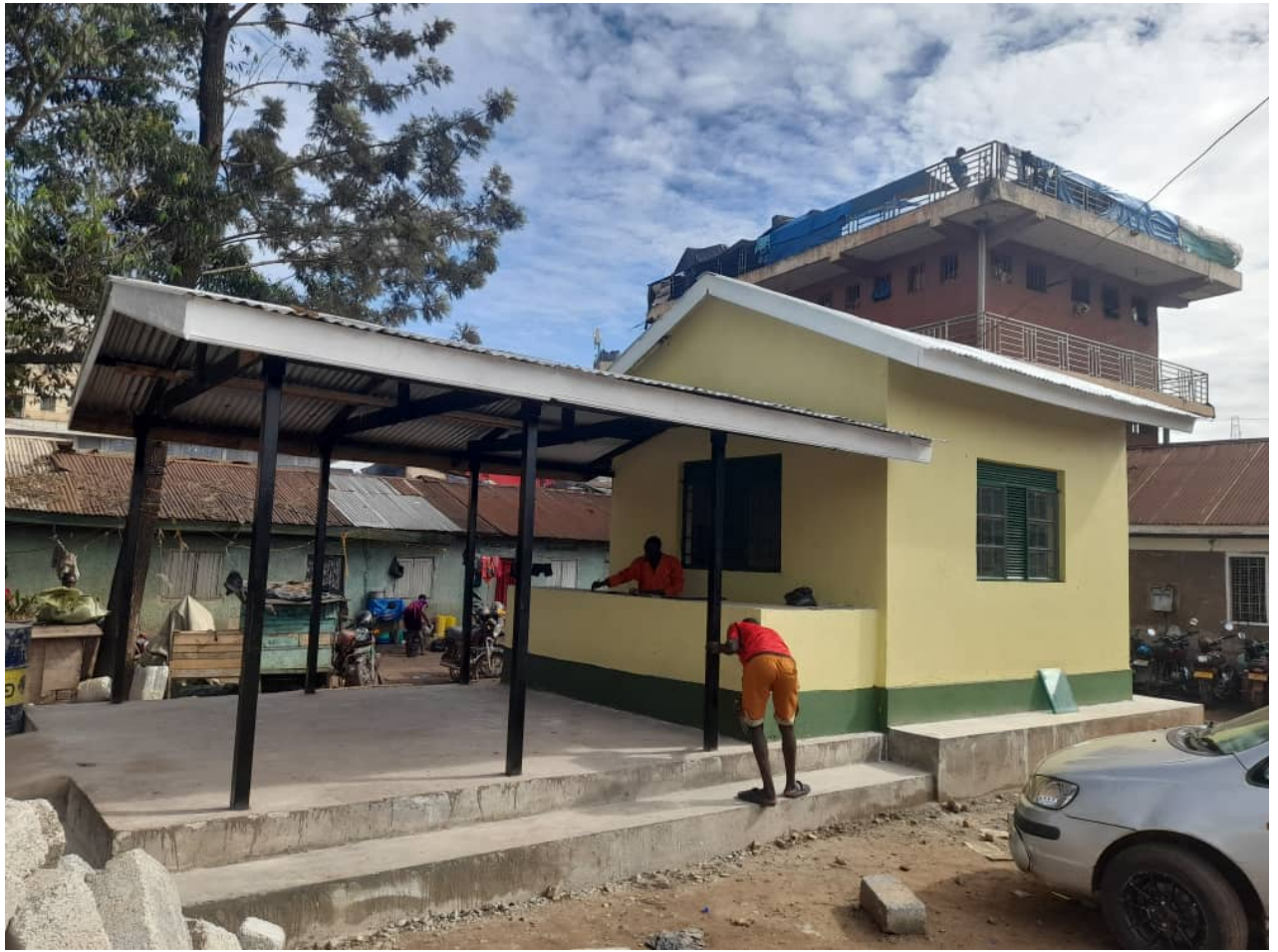
Fig. 27: Painting the exterior
