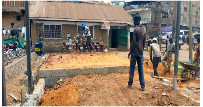
Fig. 10: Compaction of Backfill Material in Foundation
