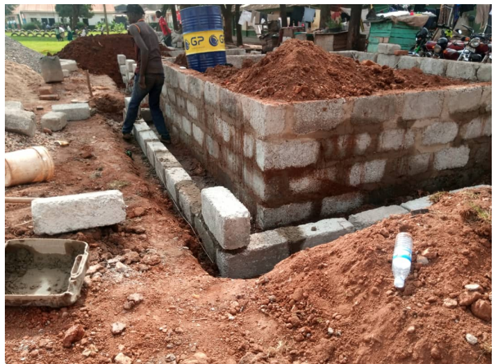
Fig. 8: Construction of Veranda walls
