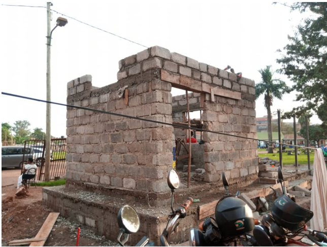
Fig. 17: Over Beam Walling
