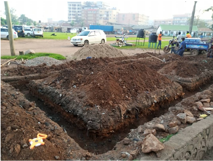
Fig. 3: Excavation for Foundation
