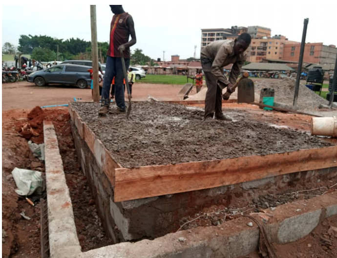
Fig. 13: Casting ground floor concrete slab
