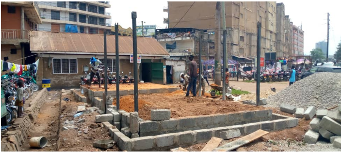
Fig. 11: Installation of Steel Column Posts for Serving Point Shade
