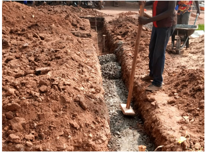
Fig. 6: Levelling and compaction of Concrete for Foundation
