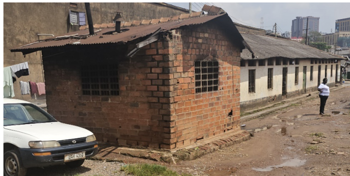
EXISTING KITCHEN HOUSE
