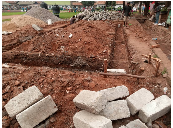
Fig. 4: Excavation for Foundation
