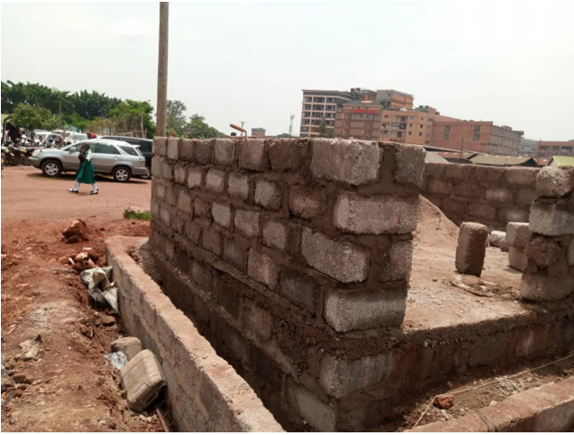
Fig. 15: Super Structure Walling
