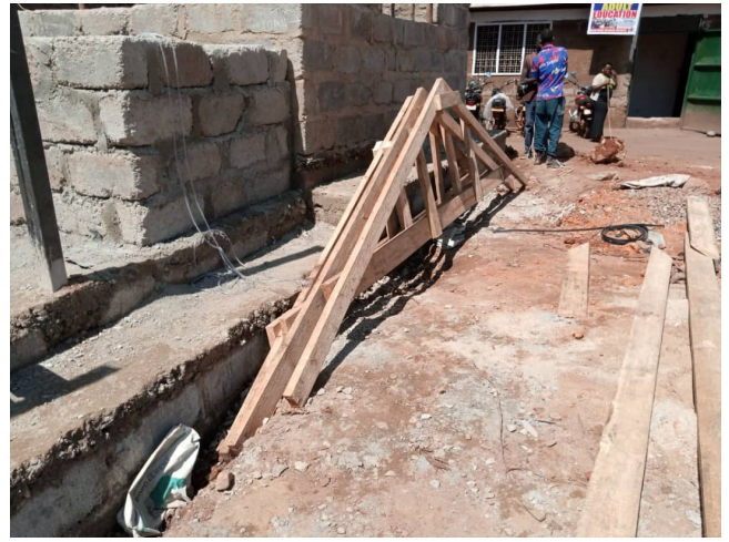
Fig. 20: Roof Truss Framing
