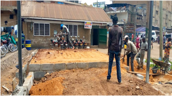
Fig. 9: Compaction of Backfill Material in Foundation
