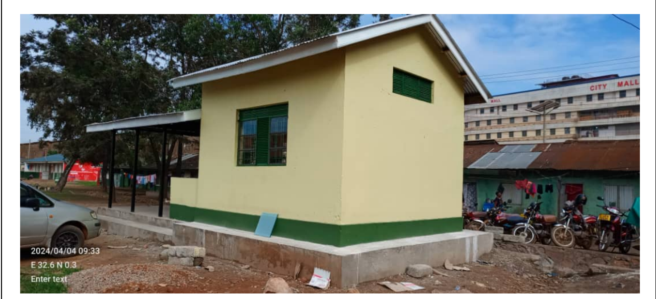
Fig. 29: Painting the exterior
