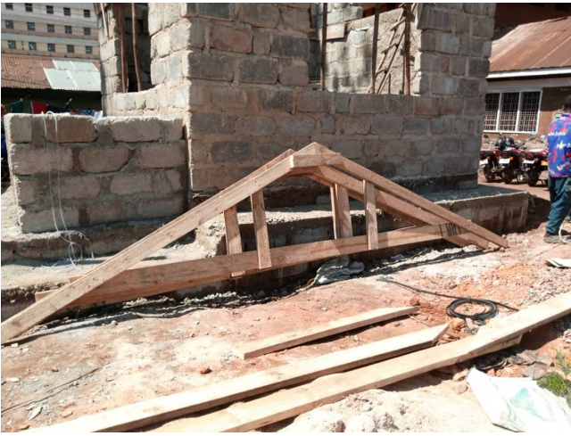
Fig. 19: Roof Truss Framing
