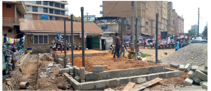
Fig. 12: Installation of Steel Column Posts for Serving Point Shade
