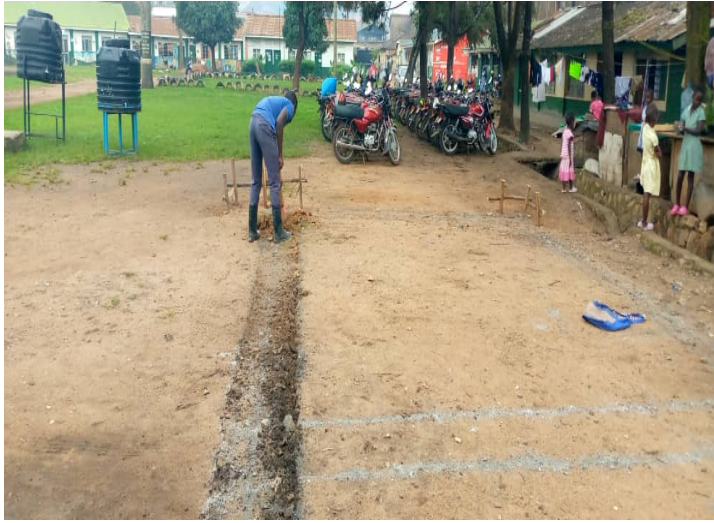
Fig. 1: Excavation for Foundation
