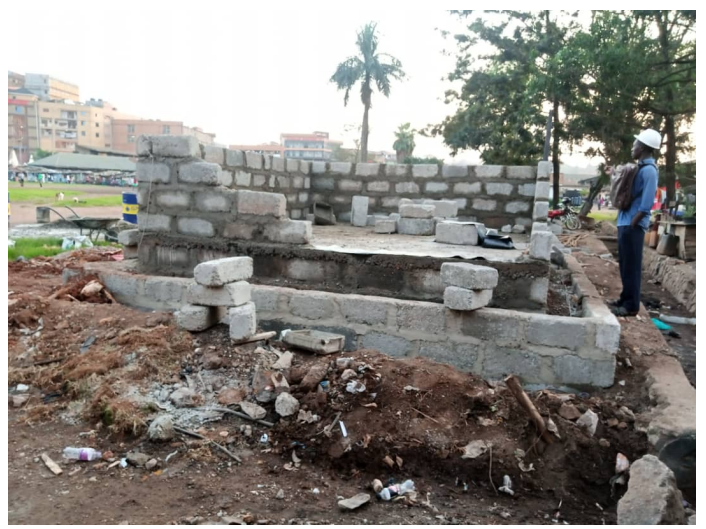
Fig. 14: Super Structure Walling
