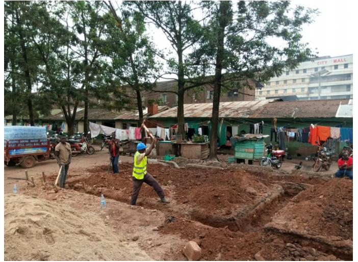
Fig. 2: Excavation for Foundation
