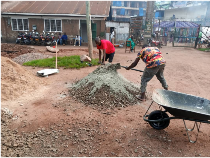
Fig. 5: Mixing of Concrete for Foundation
